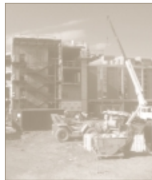
Construction of the new Cancer Center pictured here during late fall 2002.
